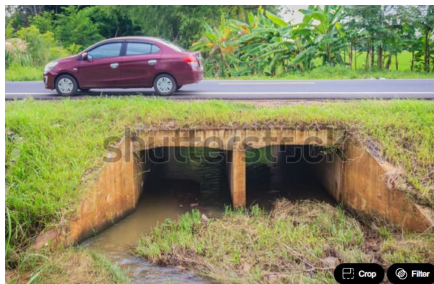
Example multi-cell box culverts
