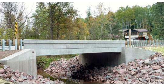
**Example Slab-Span Bridge**
