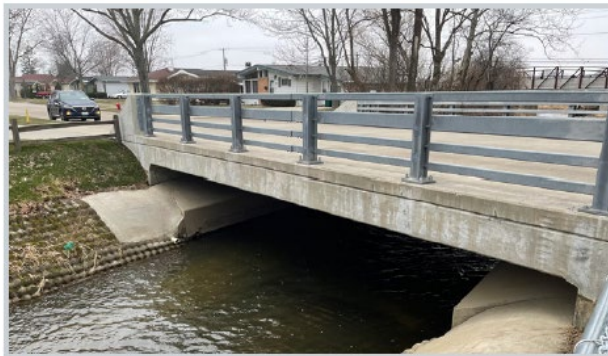
Example Concrete Slab Bridge (Selected Alternative)
