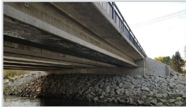
Example Prestressed Concrete Girder Bridge
